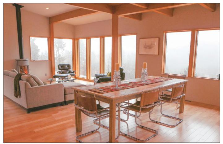
Thin-set plaster walls in environmental colors contrast with exposed timber-frame elements in the Kinnear/Mosqueda home. The ceiling above the dining area has fir beams below tongue-and-groove hem-fir decking, but the couple also wanted painted walls and ceilings in earthy colors.
