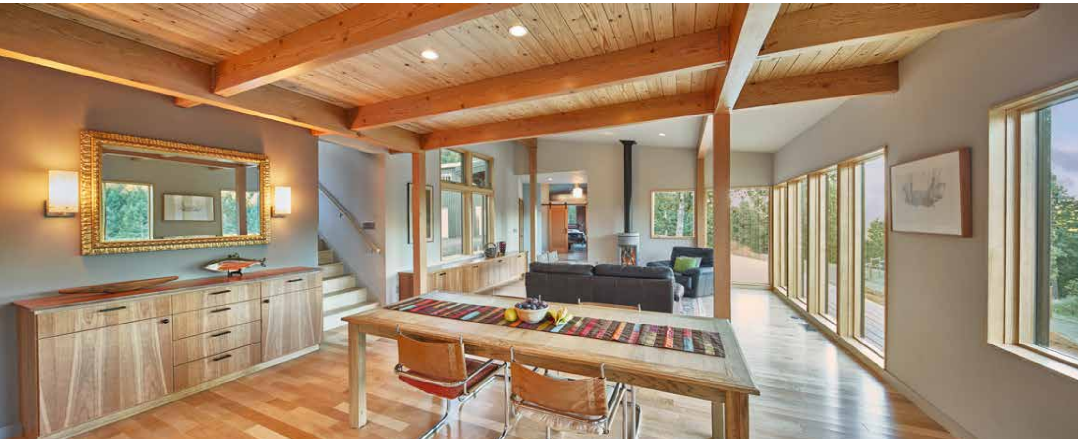
Below: A timber-framed assembly of Fir and hemlock hovers above the dining area, supporting the master suite on the second floor.
